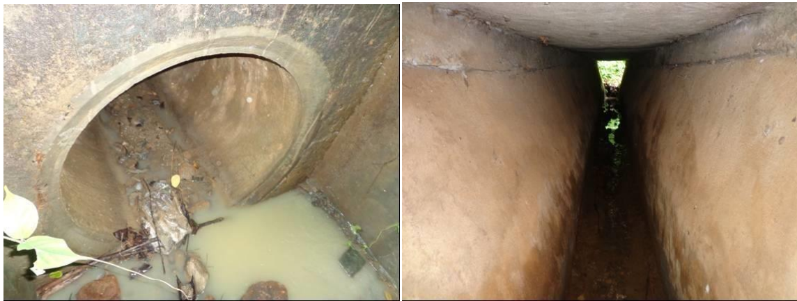
Photo 11.1 Existing Pipe Culvert (L) and Slab Culvert (R) Along NH51
