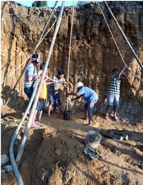
Fig-2.0 Boring in Progress,
