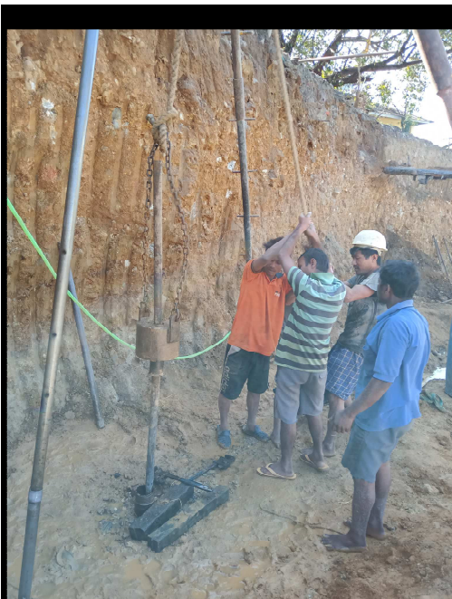
Fig-2.2 SPT in Progress
