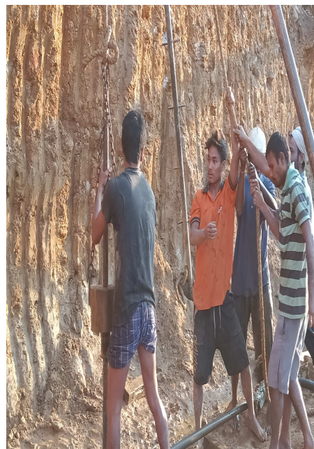
Fig-2.1 SPT arrangement in Progress
