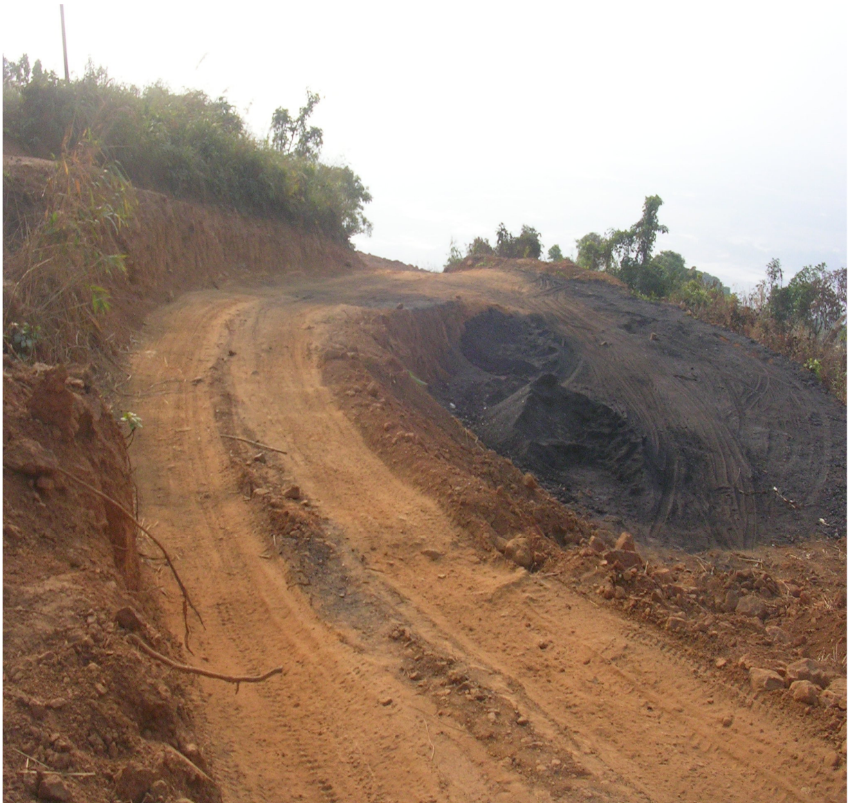
Existing Road Badly Damaged and road to coal quarry
