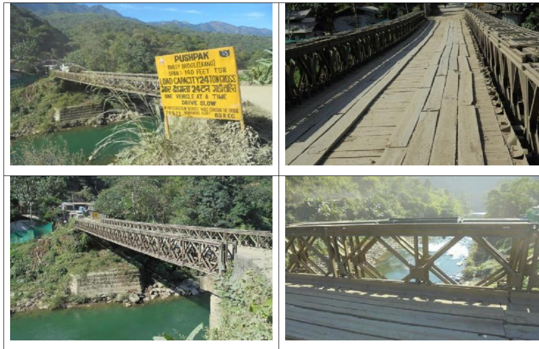
Plate – 3.1: View of existing Bridge condition near proposed Bridge location
