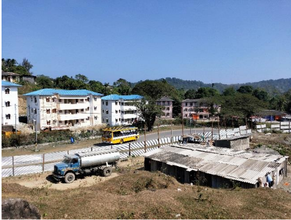
Development in the vicinity
