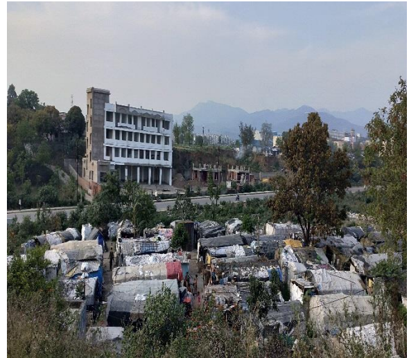
Slum encroachment at site
