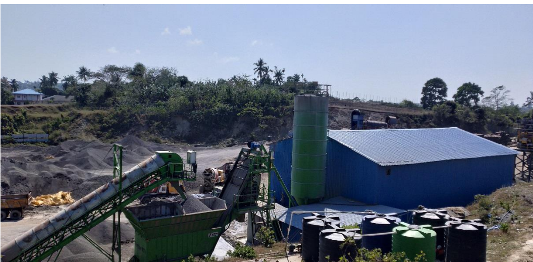
Batching Plant on Site
