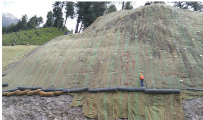
Fig. 3 – Staggered pattern of nail installation – Z-Morh Tunnel, J&K, India
