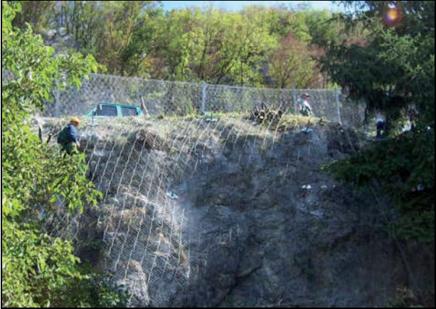
Fig. 15 – Ajdovscina, Slovenia, protection of road and residences from unstable rocks or boulders.
