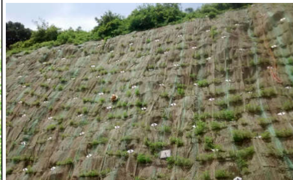
Fig. 13 – Slope Stabilization at Kiratpur-NerChowk Expressway, Himachal Pradesh
