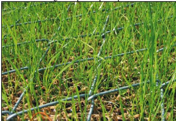
Fig. 10 – High-tensile steel wire mesh and erosion control mat
