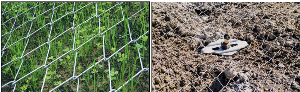
Fig. 1 – High-tensile wire mesh for slope stabilization (left) and special spike plate to actively pressing the high-tensile steel wire mesh against the slope surface (right)
