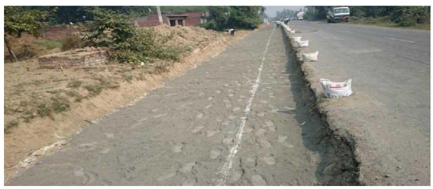
•Line marking was done at 2.4 meters from toe line for Operator's guidance
