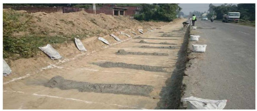
•Grid were made on the prepared sub-grade top to spread cement
