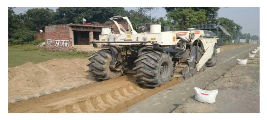
WR2400 : Wirtgen stabilizer and recycler In process of mixing existing prepared sub-grade top with pre spread Cement .
